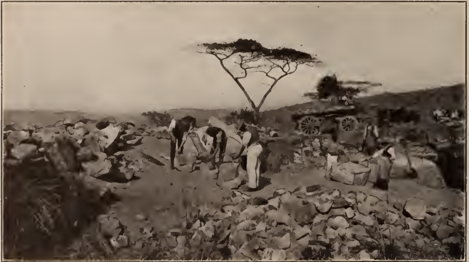
AT THE QUARRY.—ULU BOYS LEARNING TO MAKE GOOD FOUNDATIONS
